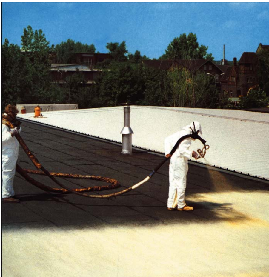
Fig. 37: Thermal insulation and sealing in one operation
